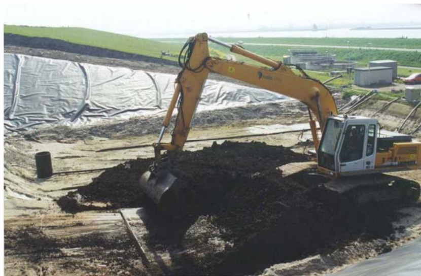
Figure 4-45. Construction of the Nauerna pilot-scale landfill (van Zomeren and van der Sloot, 2006b).
